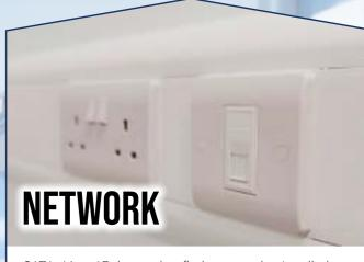
CAT6, 6A or 6E data outlets flush mounted or installed within trunking, cabled back to network patch panel for client connection to host building server. Can also be incorporated into the EMS and BMS.
