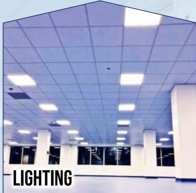
Powder-coated steel light units, flush mounted into the ceiling panels with drop-down hinged diffuser. Also available as surface-mounted aluminium LED batten luminaires for laboratories. Activation by switch or PIR (passive infrared) sensor. Lights can be UV filtered for photo-sensitive processes.
