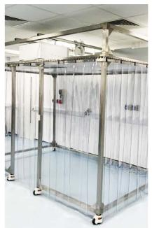
obstacle for Guardtech. The team opted to use slimline Fan Filter Units in order to create the tallest internal ceiling that could be achieved for the Isopods.
